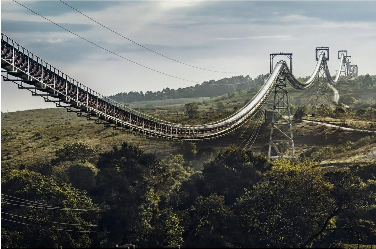
© BARROSO-MG, 27/08/2015 SEMPERTRANS Photos of the Flying belt system installed at Holcim Barosso Cement Manufacturing Plant. The flying belt system was ordered by Holcim at Agudio, which Sempertrans delivered the Conveyor Belt. Flying belt is an aerial transport system for bulk materials on ropes with conveyor belt. Foto: Bruno Figueiredo / çrea de Servi•o
